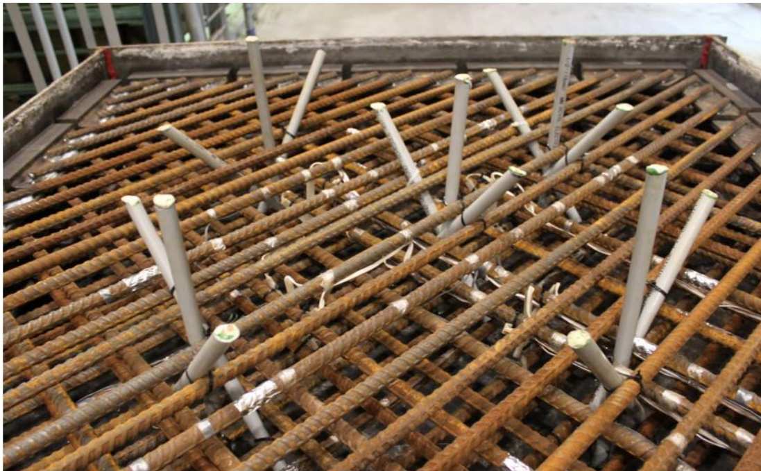
Figure 21. Out-of-Plane Instrumentation in Reinforcement Cage
