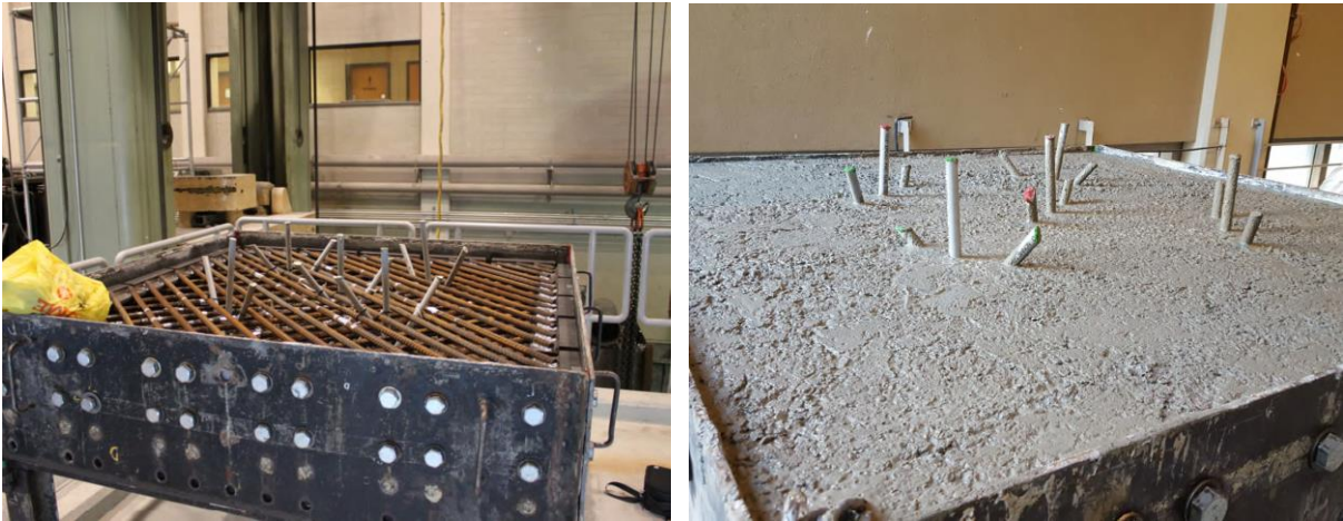
Figure 3. Casting Reinforced Concrete Shell Specimens
