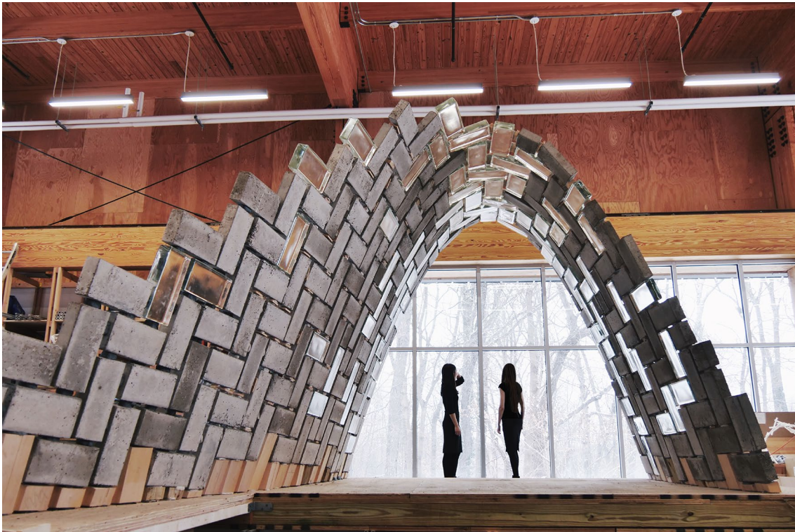
Fig. 1 Finalised prototype of robotically assembled brick vault
