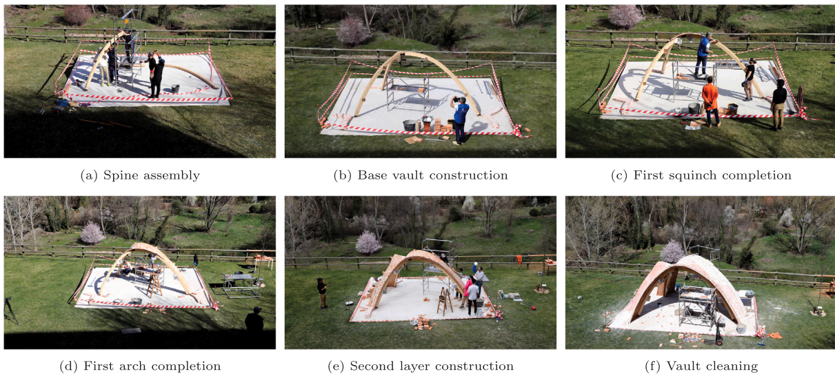
Fig. 17. Timelapse of the key steps of the construction process.
