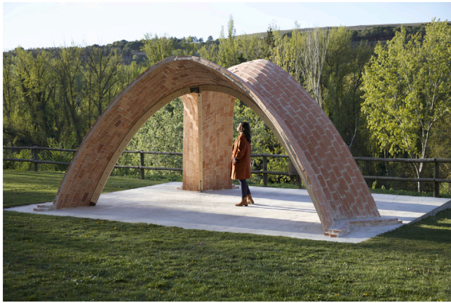
Fig. 1. The innixAR prototype of a masonry vault demonstrating how to design and build for minimal falsework, leveraging 4D funicular design, thin-tile vaulting, loxodrome tessellation, augmented reality, and prefabricated spine.
