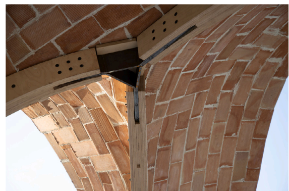
Fig. 13. Central connection detail with steel node, timber spine legs, and masonry squinches.
