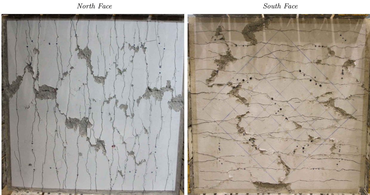
Figure 5.5: ES2 at Failure (Black Lines = Cracks)
