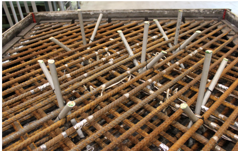
Figure 3.27: Out-of-Plane Instrumentation in Reinforcement Cage
