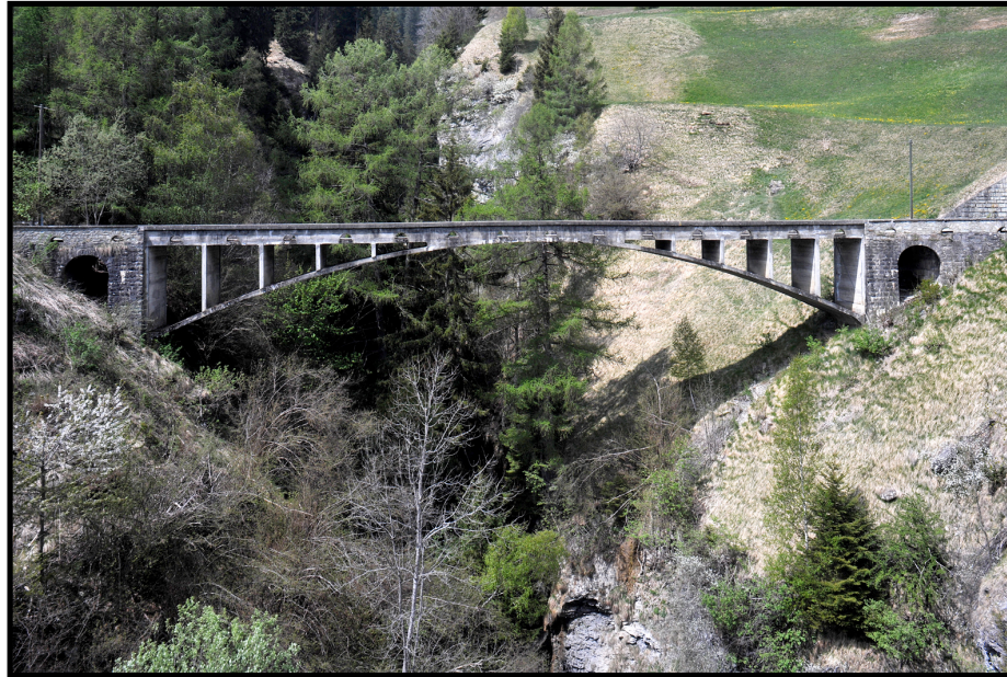
Figure 5. The Valtschielbach Bridge (1925) in Donath, Switzerland (Kleis, 2011).
