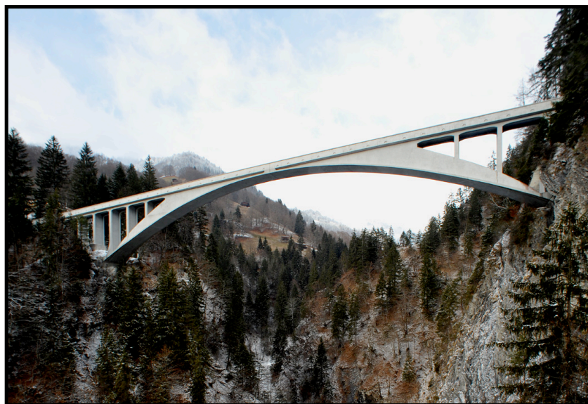
Figure 3. The Salginatobel Bridge (1929) over the Salgina Brook in Schiers, Switzerland (Kleis, 2011).
