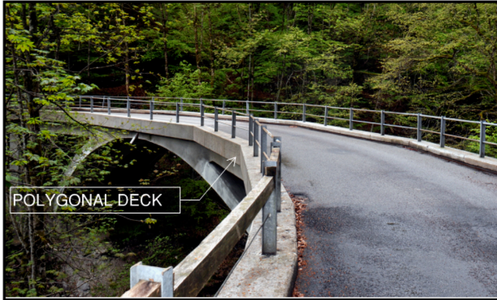
Figure 7. The Ziggenbach Bridge (1923) in the Wägital Valley, Switzerland (Kleis, 2011).
