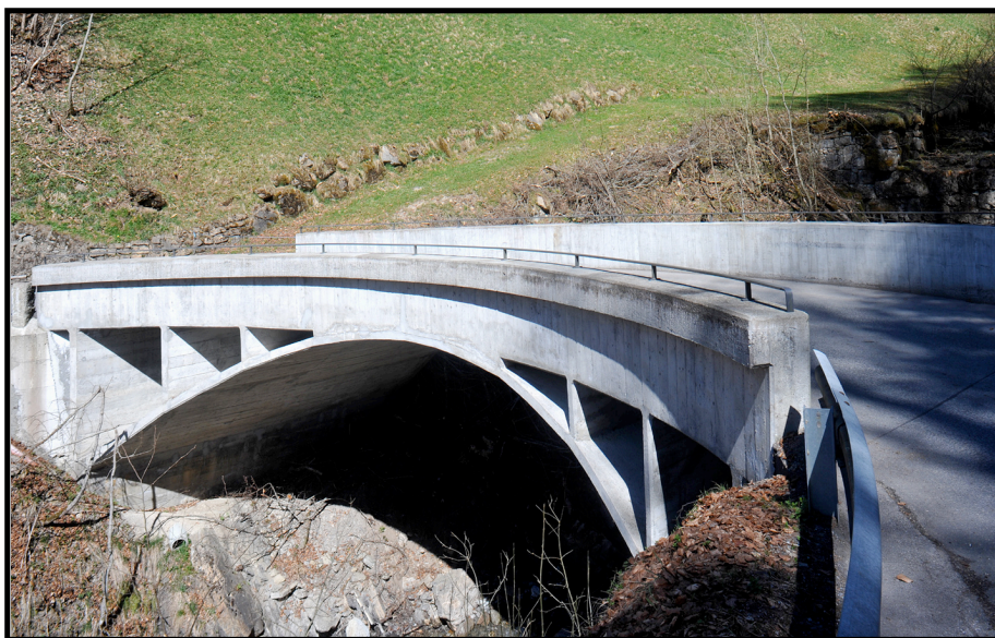
Figure 8. The Bolbach Bridge (1932) in Habkern, Switzerland (Kleis, 2011).
