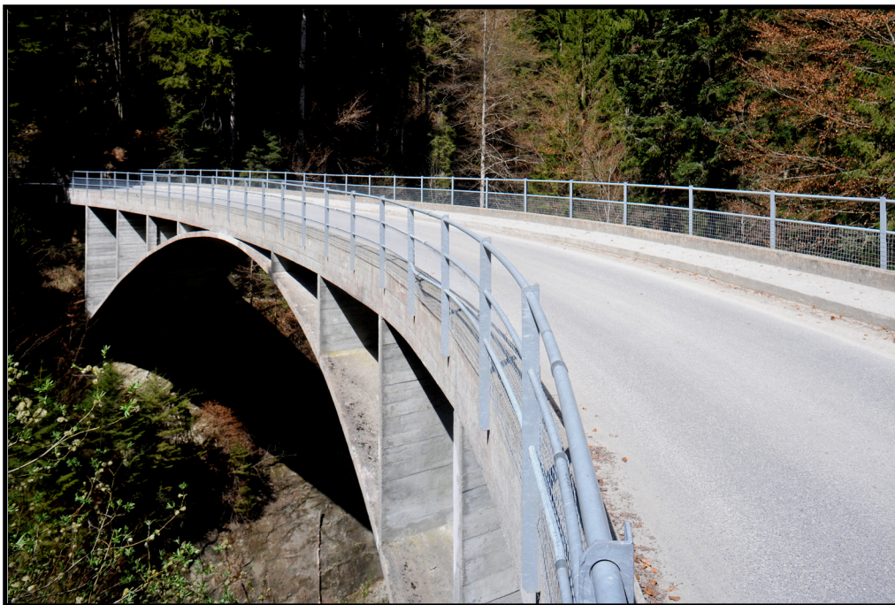
Figure 9. The Schwandsbach Bridge (1933) in Hinterfultigen, Switzerland (Kleis, 2011).
