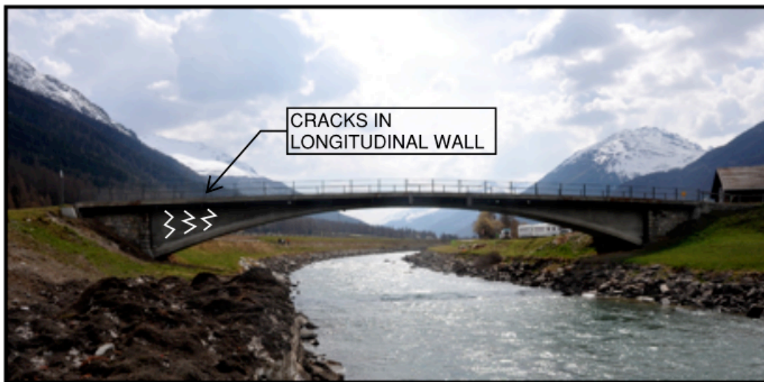
Figure 1. The Zuoz Bridge (1901) over the Inn River, Switzerland (Kleis, 2011).
