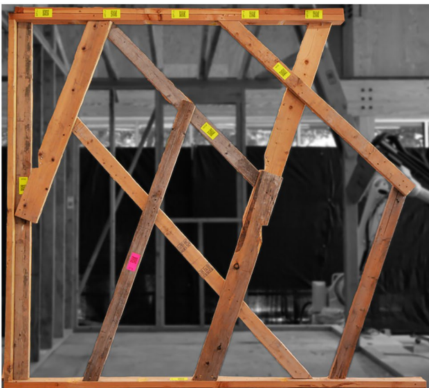
(b) Elevation of the finished West wall reassembled into a lattice structure.
